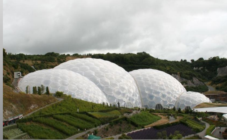
example: Eden Project, Cornwall, UK constructed with ETFE cushions
